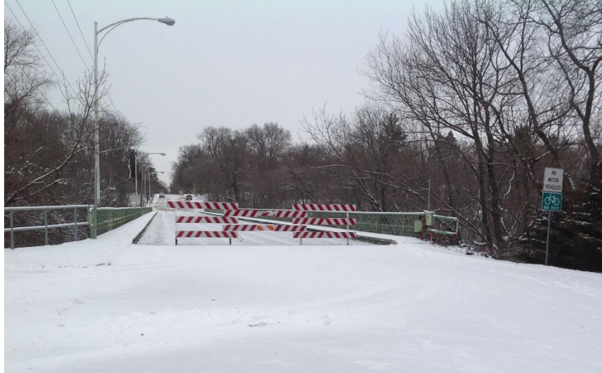
Figure 11 Closed Centennial Bridge in Crapo Park, Burlington, Des Moines County
